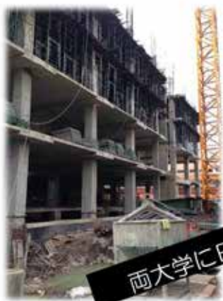
建設中のThammasat University Hospital
